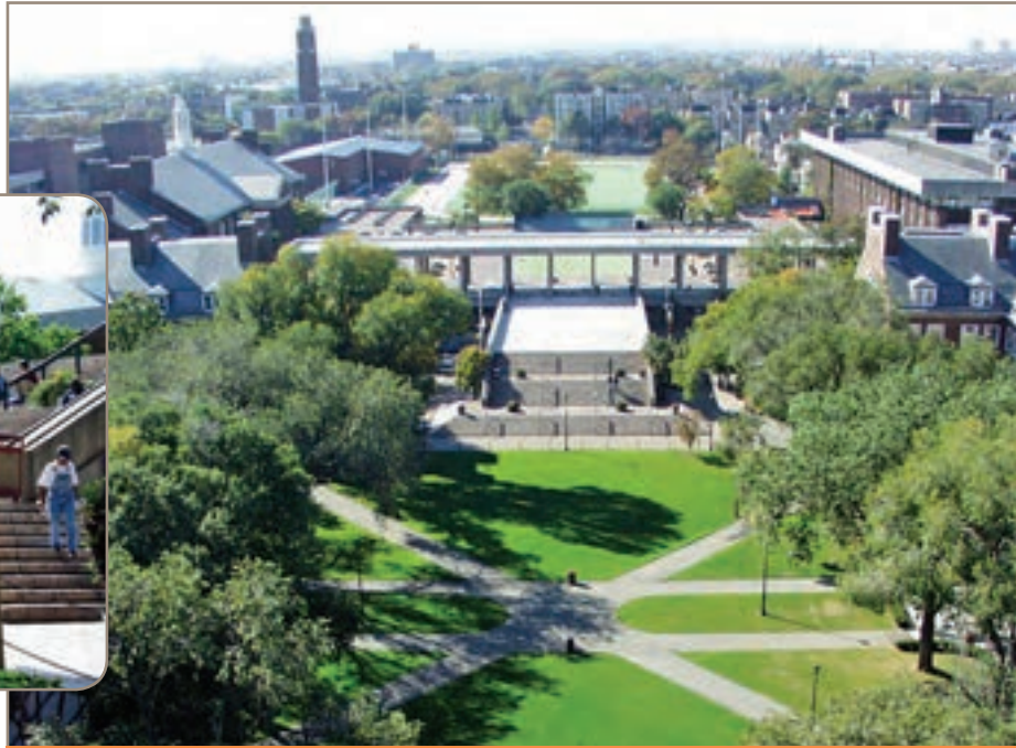
Plaza Building Overpass 1980s
